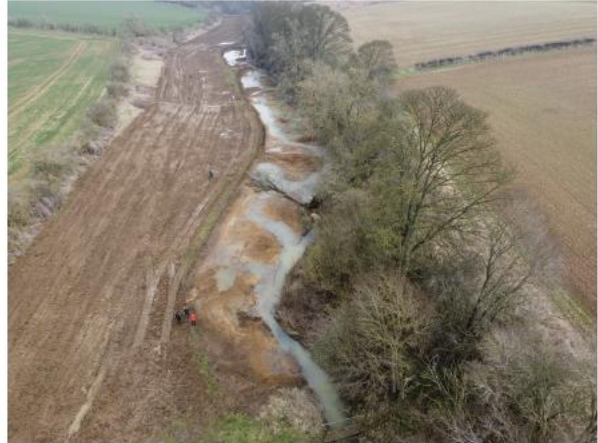
View of top section of site after works
