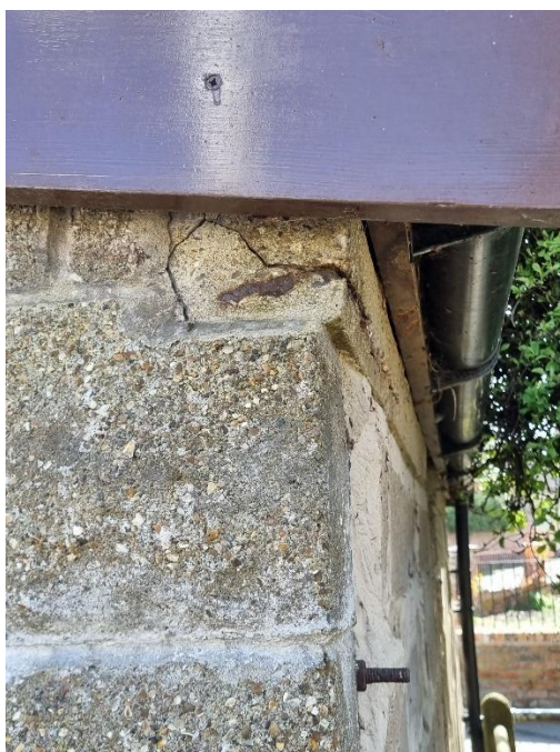
Smaller crack
